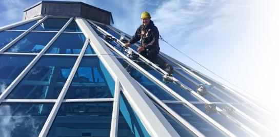
Designed to meet the requirements of the commercial and light industrial sectors, our glazing bar system can be used with multi-wall polycarbonate sheets, 6mm single glazed units and double glazed units.
